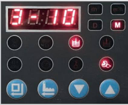
With the help of the UP and DOWN keys, indicate the brine suction time of your water softener (table 2). Press "menu / confirmation" to confirm.
